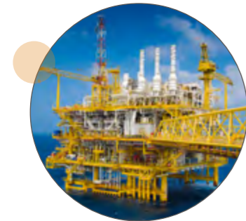
B Protect operations on offshore platforms
